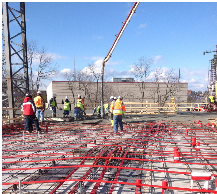
Figure 1.6. Structural Post Tensioned Deck
