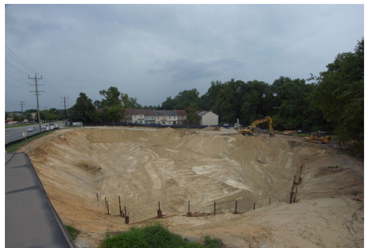
Figure 1.4. Excavation & Earth Retention
