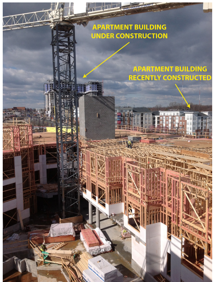
Figure 4.1. Nearby Apartment Buildings
