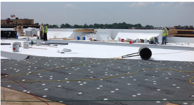
Figure 1.8. TPO Membrane Roof
